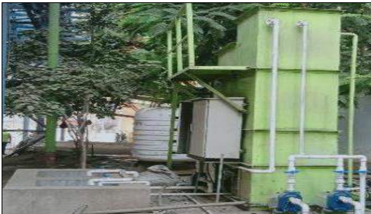
Sewage Treatment Plant Installed at CCR Area (Capacity: 5 KLD)
