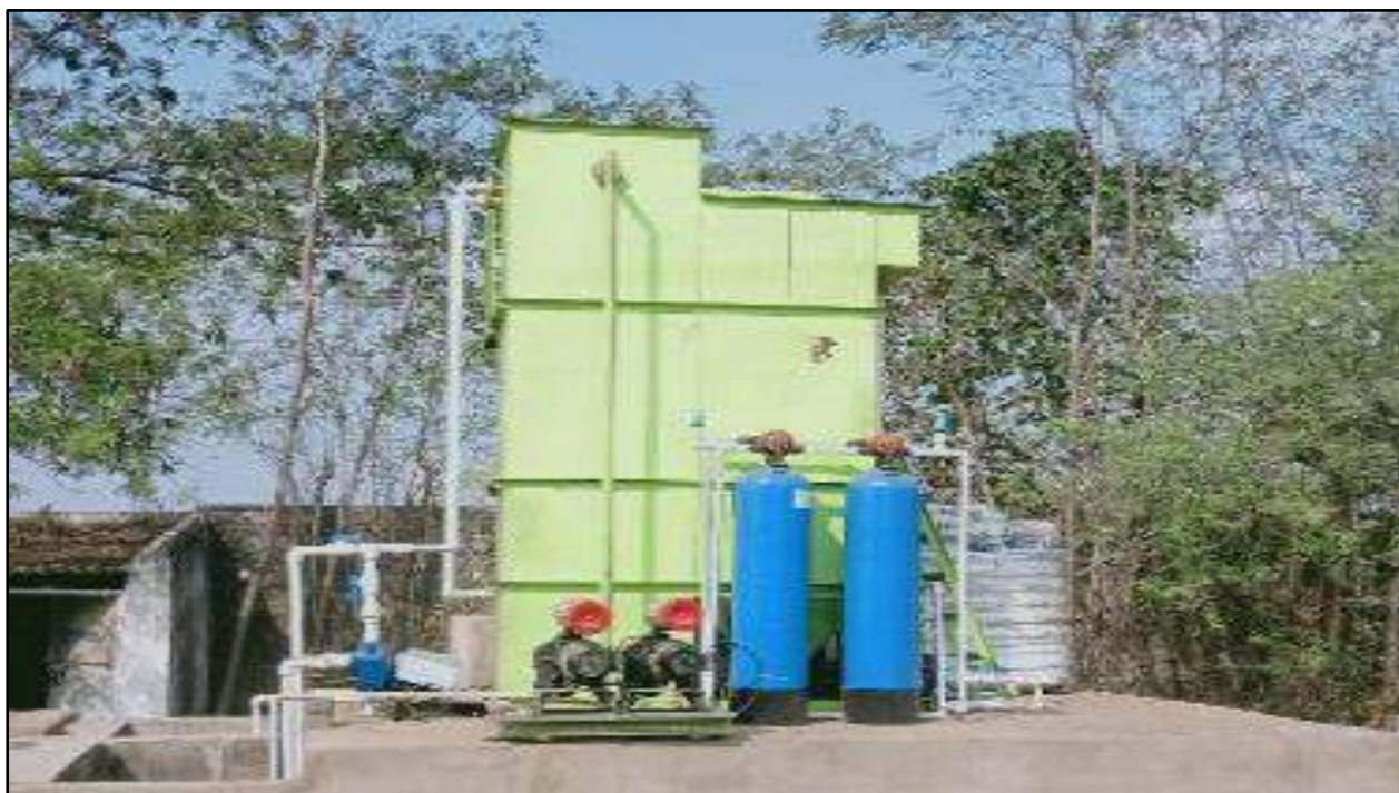
Sewage Treatment Plant Installed at Packing Plant Area (Capacity: 5 KLD)
