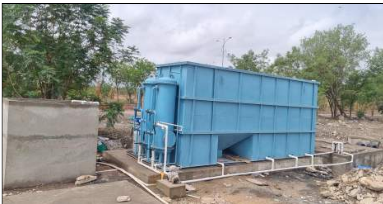
Sewage Treatment Plant Installed near Staff Colony (Capacity: 75 KLD)
