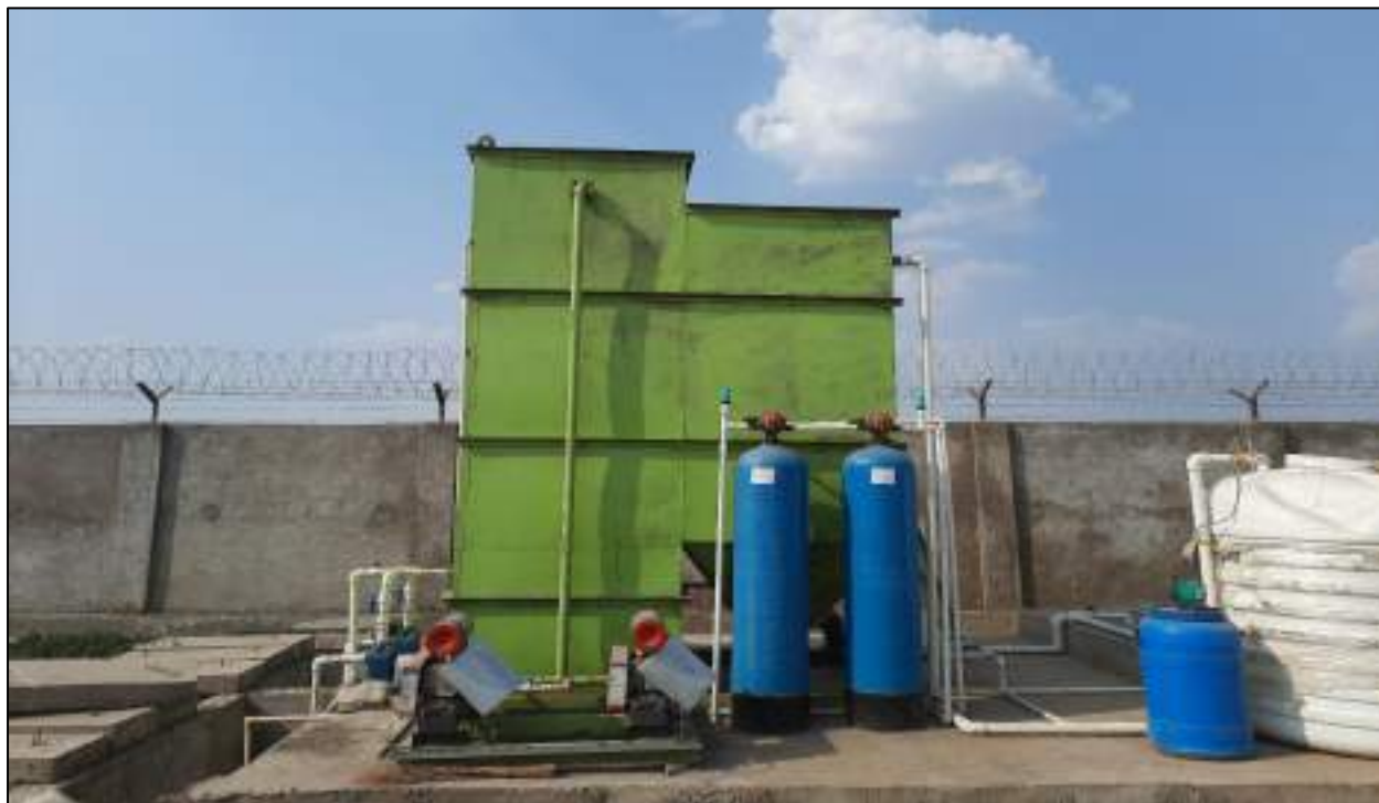
Sewage Treatment Plant Installed at Temporary Hutment Area (Capacity: 20 KLD)
